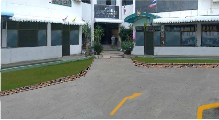
Proposed green areas near the steps maybe with seating area and plants
