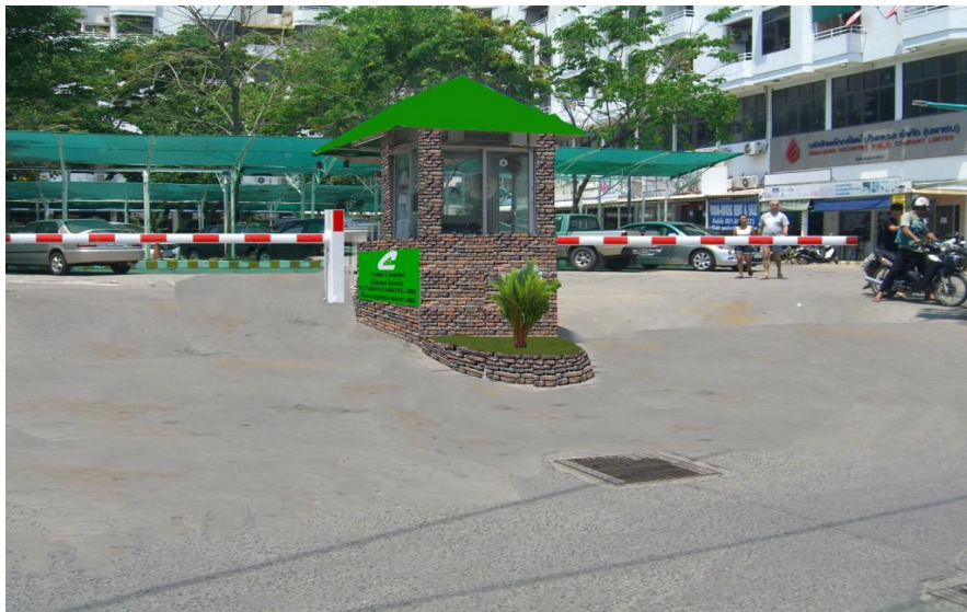
New security box and barriers
